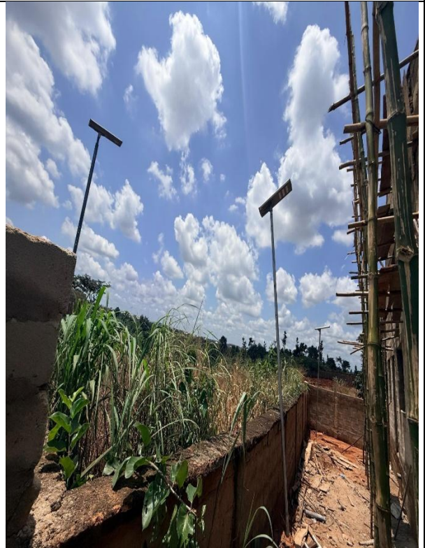
Plate E4: Site side view also showing solar provisions
