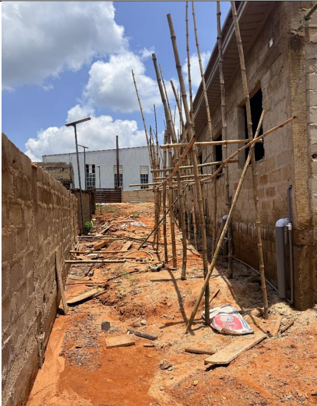
Plate E3: Site Rear view
