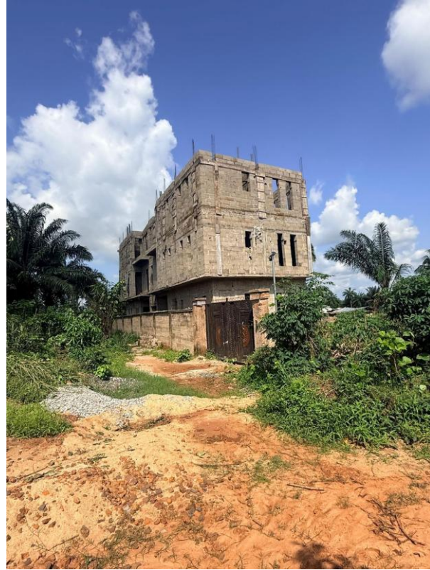
Plate A1: Front view of the building from the approach path, showing the perimeter fence, gate and the surrounding
