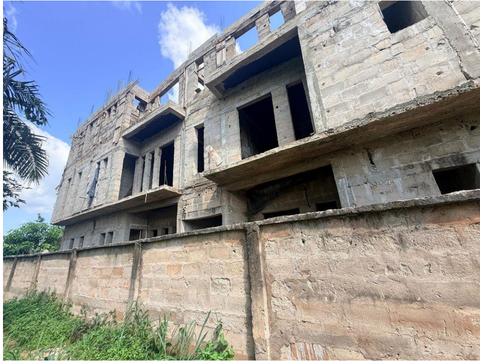
Plate A4: Close view of the building carcass, showing block walls to roof level, exposed reinforcement starter bars, and unfitted window and door openings
