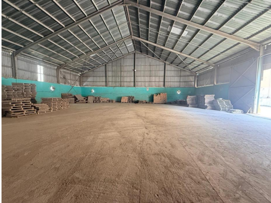
Plate 2.4: Interior of the Storage Warehouse with Palletised Stock
