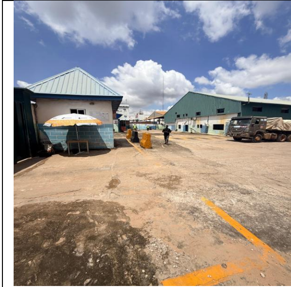
Plate 2.2: General View of the Depot Yard, Office Block and Truck Bay
