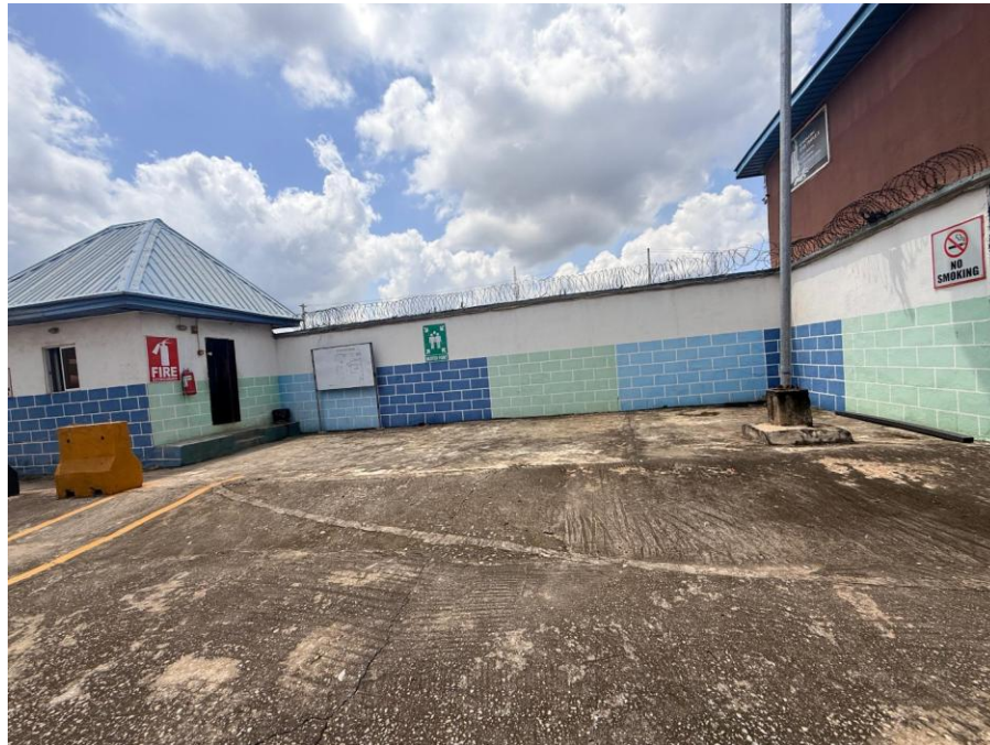
Plate 2.1: Perimeter Wall Showing Fire Point and Muster Point Signage
