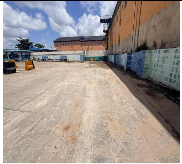
Plate A.2: Yard Corner Showing Painted Parking Blocks
