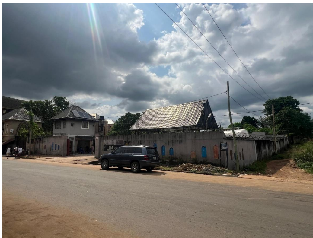
Figure 9. Picture showing alternate view of the facility
