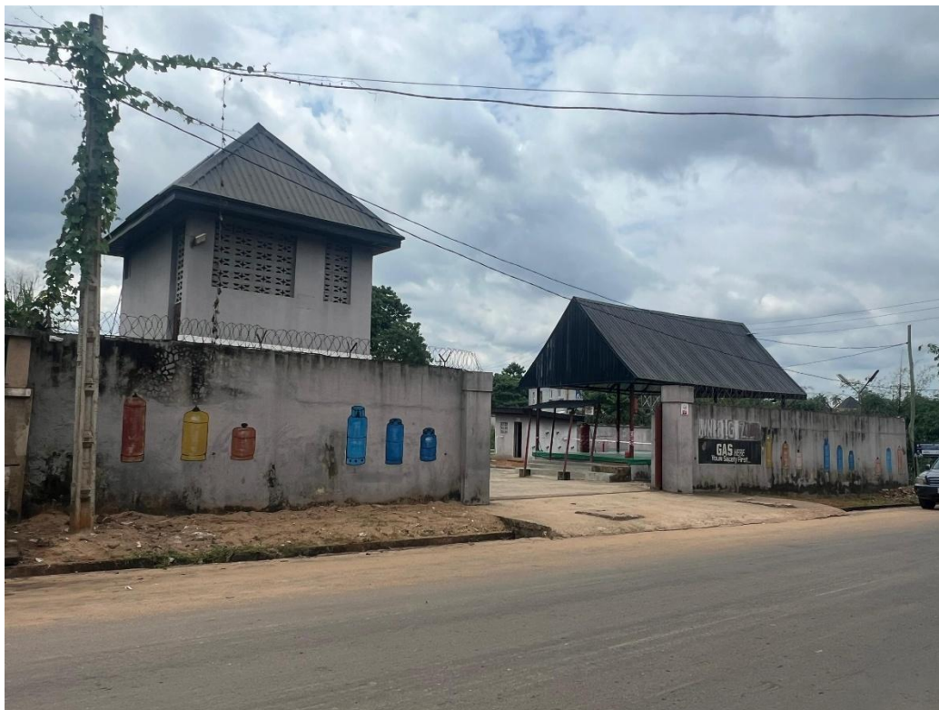
Figure 8. Picture of the facility entrance from across the road
