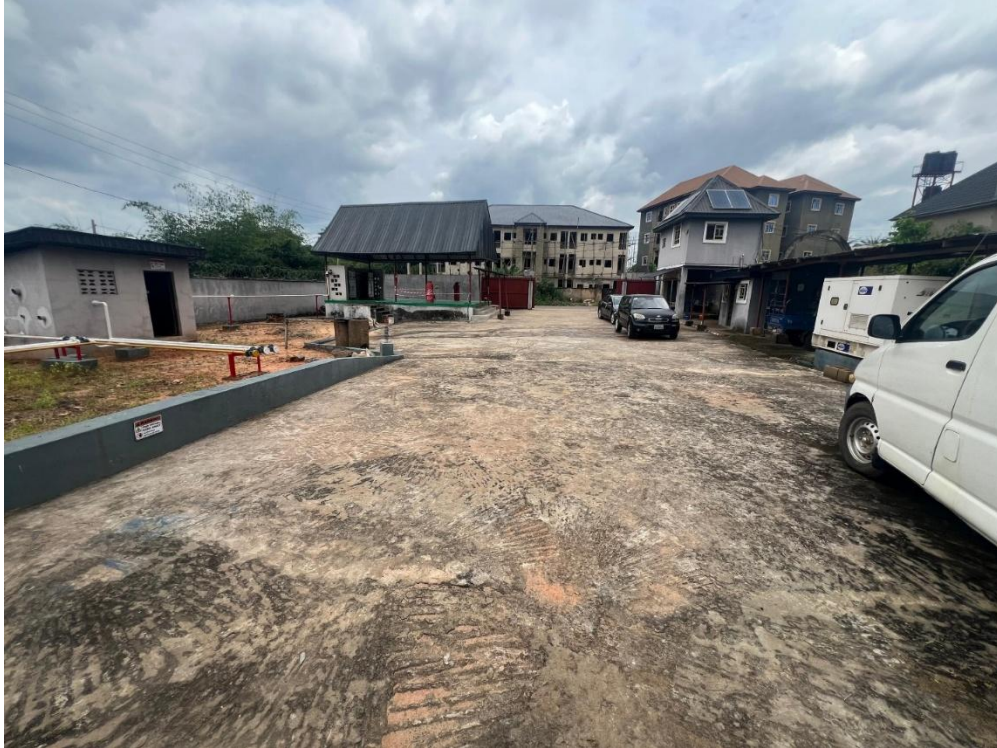
Figure 2. Picture of the compound and entrance gate
