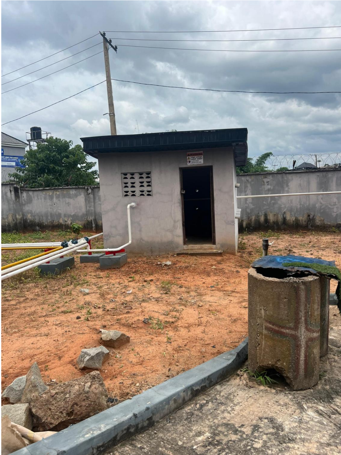
Figure 6. Control and utility house
