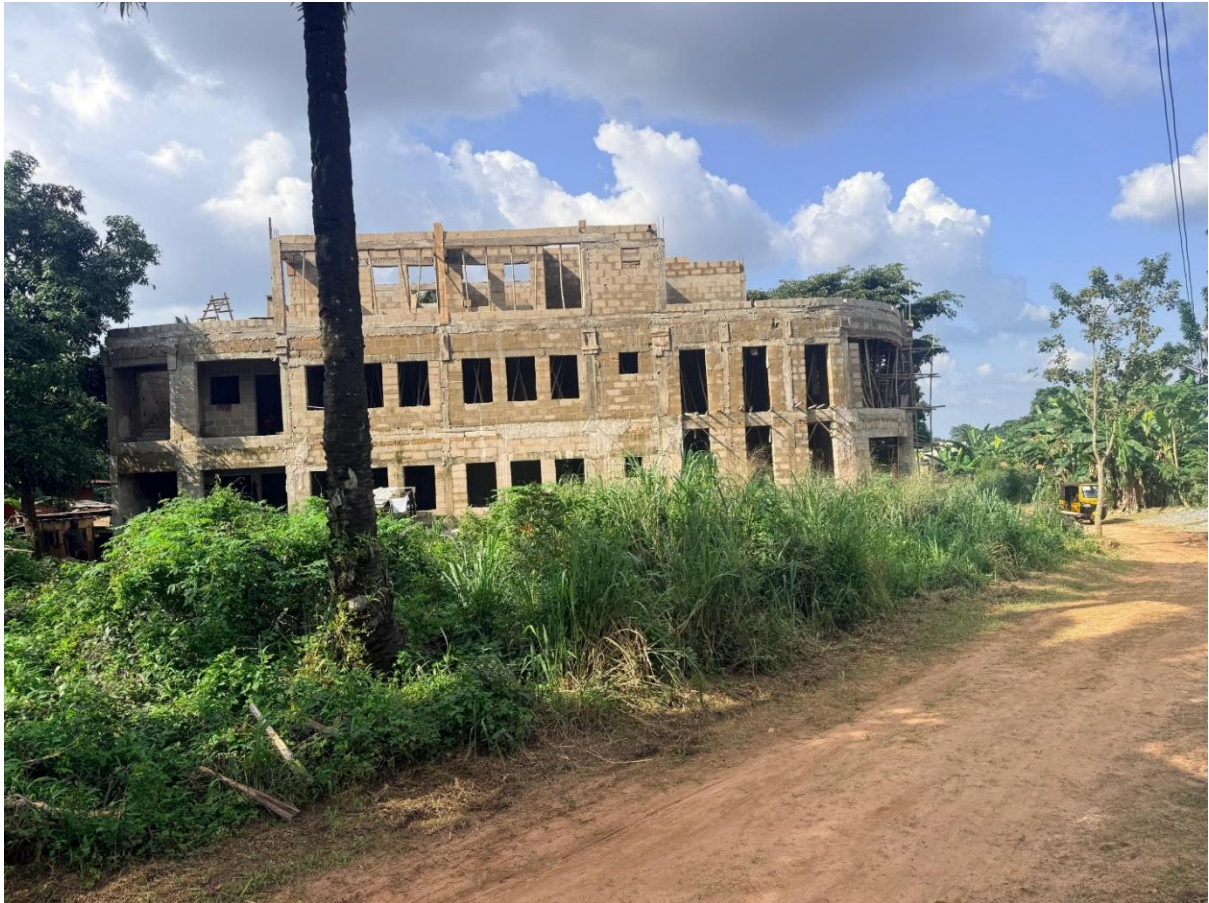
Plate D3: access picture of the site
